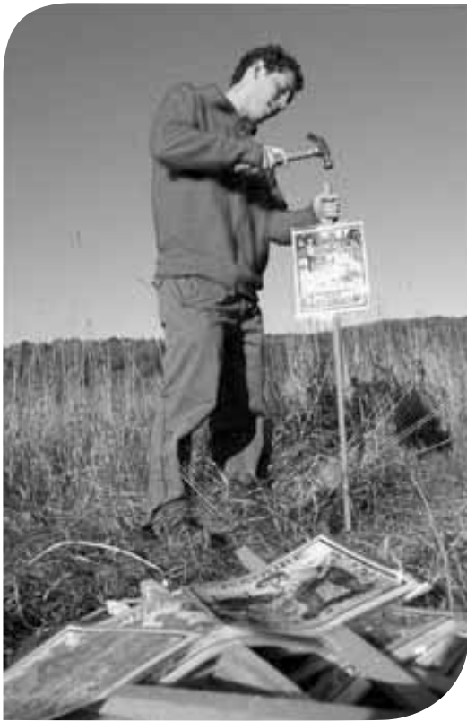
Larry Clarfeld, an AmeriCorps member, installs a StoryWalk station along a walking path at the North Branch Nature Center in Montpelier in November.
